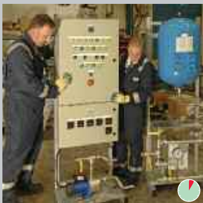
Control module and pressurisation module positioned in boiler plant room 5 mins
