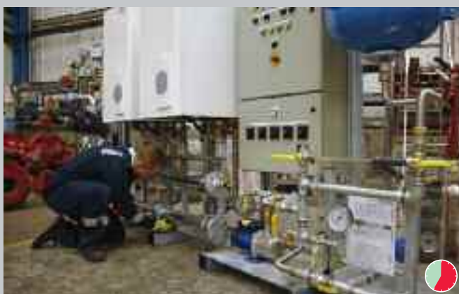
Additional boiler modules installed NB: Approximately 10 mins per module 35 mins
