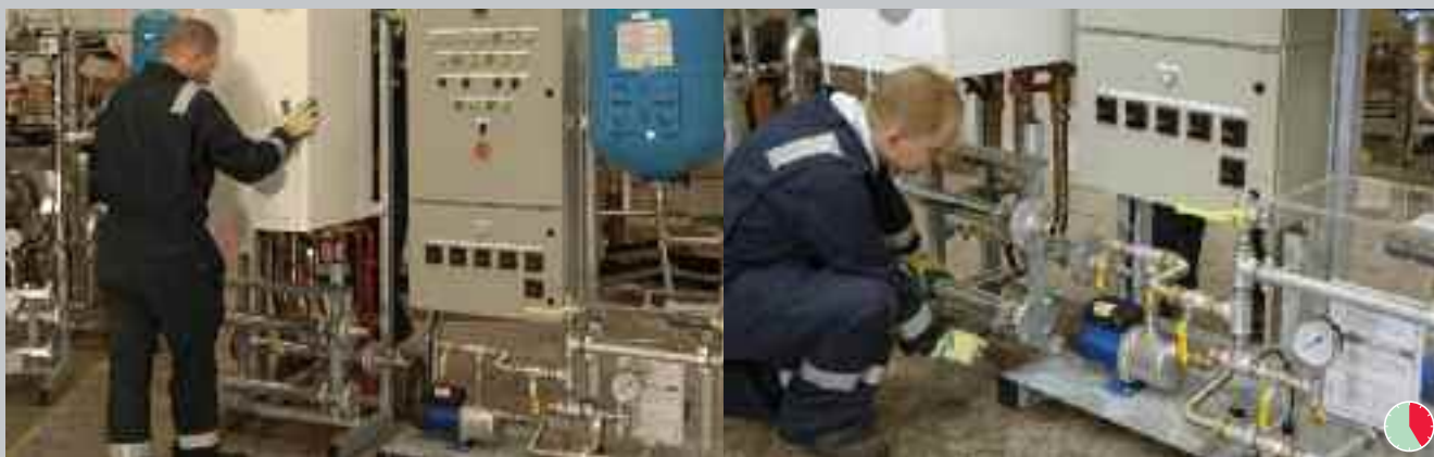
1st boiler module connected to control module 25 mins
